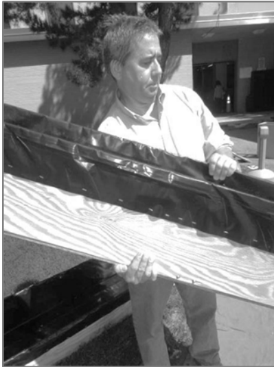
Exhibit 17. Showing how to hold a chute for the pour.
